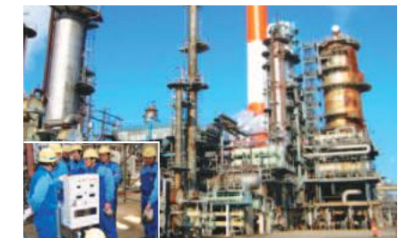
Refinery turbine lubricating oil (SRC-814-15V; explosion proof)
